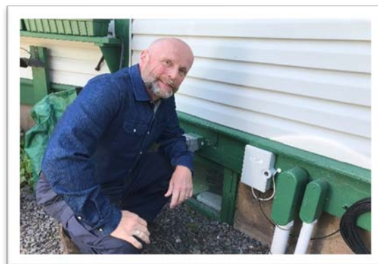
Sandy MacKay is beside the data utility box that is connected to the outside of your home. This is the first step to getting fibre to your home.
