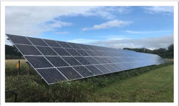
Fossil Farms is powered by 80 solar panels located near the entrance of the property.
