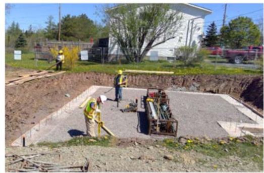
Dave Graham and volunteers Meghan Bragg and Tyler Brimicombe levelling crushed rock for basement floor. (May 20)
