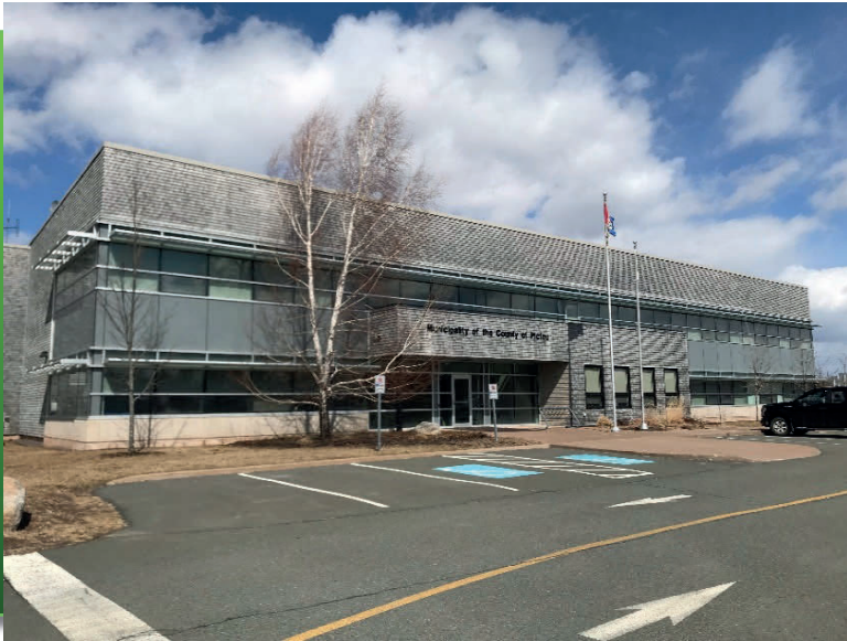
Administration Building for the Municipality of Pictou County
